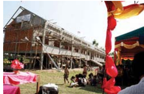
AAfC school under construction in Prek Koy, rural Cambodia
